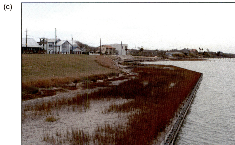
Figure 19. Photographs of shorelines protected by (a) low seawall at Goose Island State Park on the northern shore of Aransas Bay, (b) riprap and a low concrete bulkhead at Seadrift on the northern shore of San Antonio Bay, and (c) a low bulkhead and vegetation at Bayside on the southwestern shore of Copano Bay.
