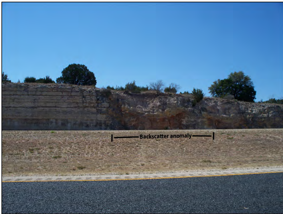
Figure 2.11 (a) Example 1 of surface anomaly that can backscatter surface waves. (b) Example 2 of surface anomaly that can backscatter surface waves. Both examples are in road cuts through a carbonate surface layer on Interstate 10 east of our study site.
