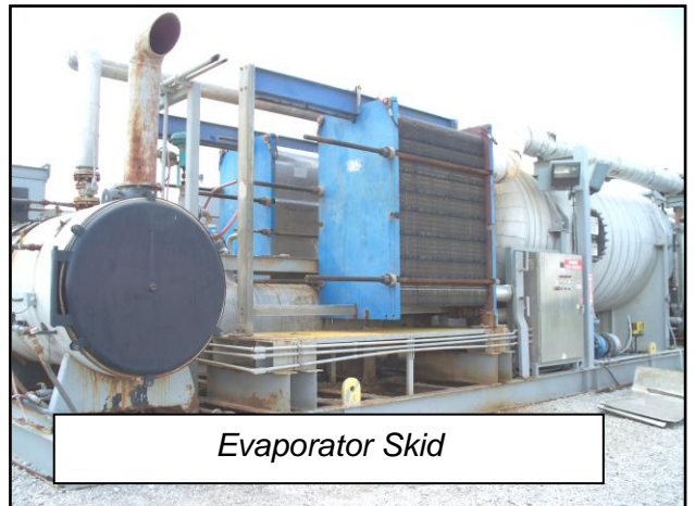
Photo 7-4: Evaporator Skid
